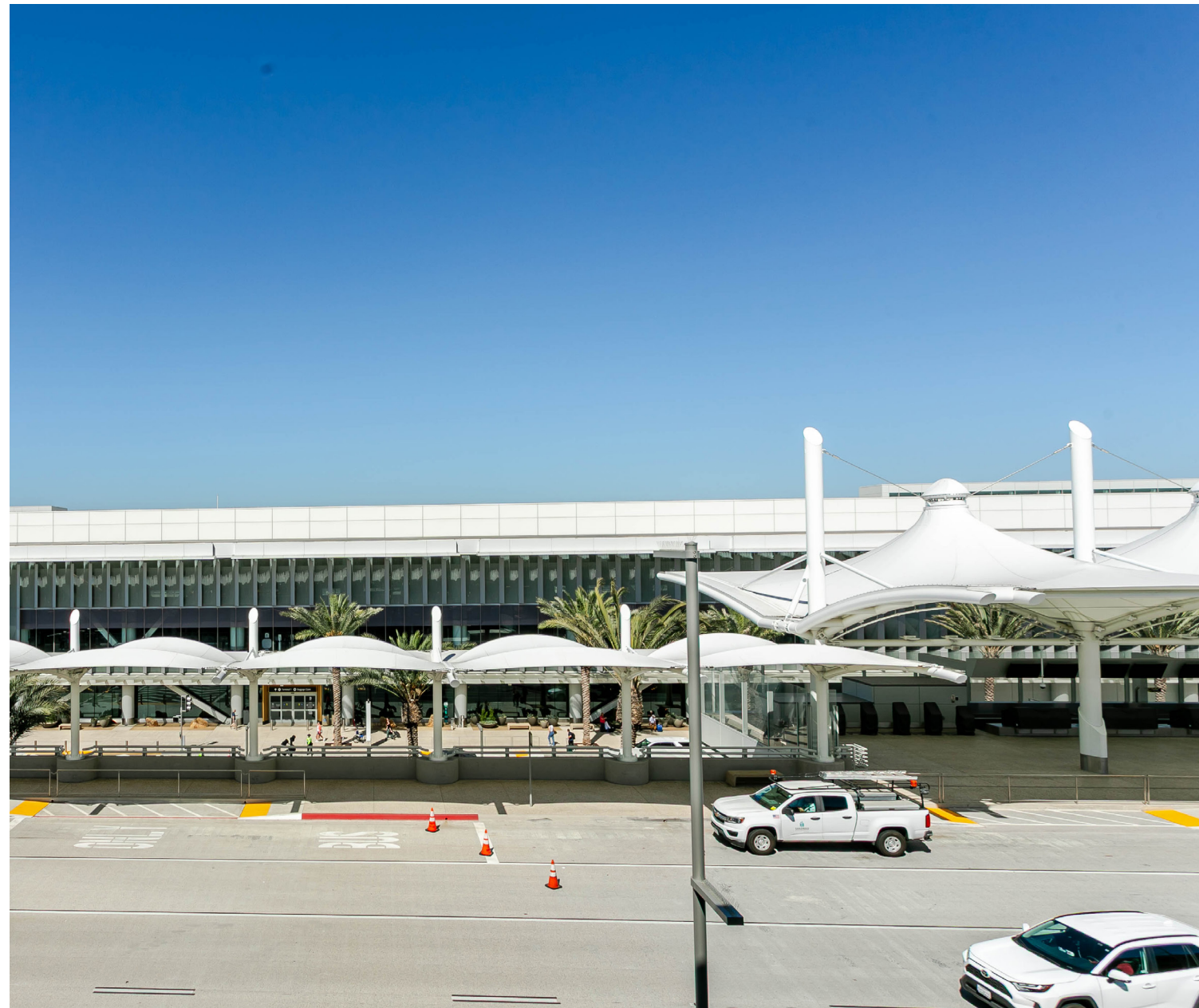
Elevated Departure Roadway of the NT1 at San Diego International Airport, designed to enhance passenger experience and operational efficiency.
