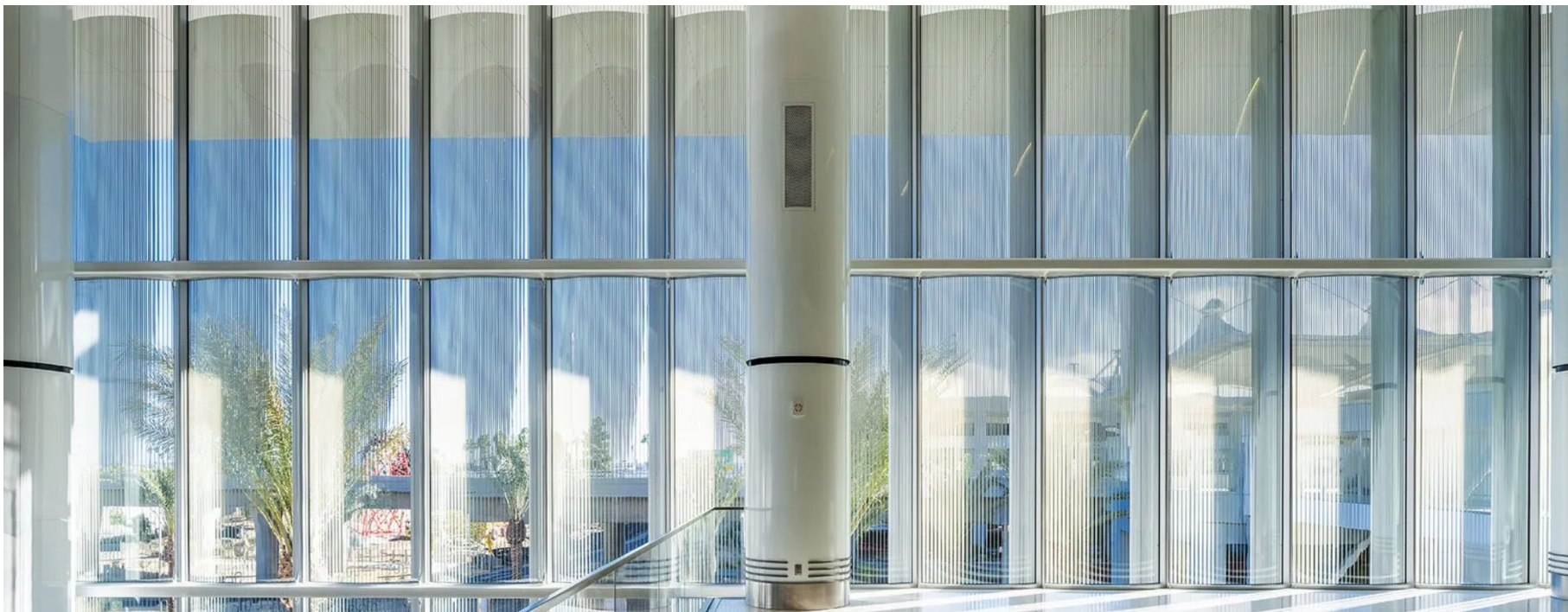
Luminous Wave, the terminal’s glass façade designed by artist James Carpenter, features 537 curved, fritted glass panels that maximize natural daylight.
