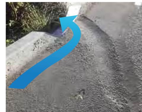
**Figure 4-3.** A runnel directs stormwater flow, San Juan Island, WA.
