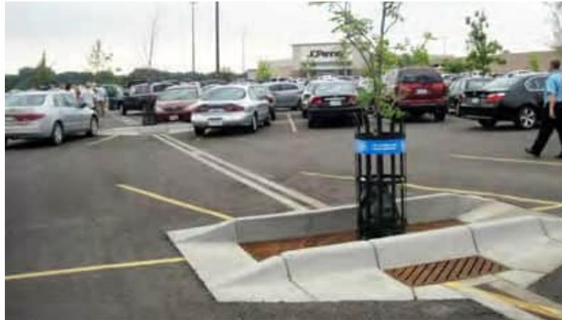
Trees are planted in groves connected by trenches in this parking lot at the Maplewood Mall, MN. Tree trenches extend 8 to 12 feet wide and 4 feet deep for a total of 1 mile in length. Angled curbs were designed to allow snow plows to roll smoothly over them.
