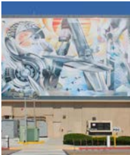
2 Javi 'WERC' Alvarez SAN Building Exterior (pre-security)
