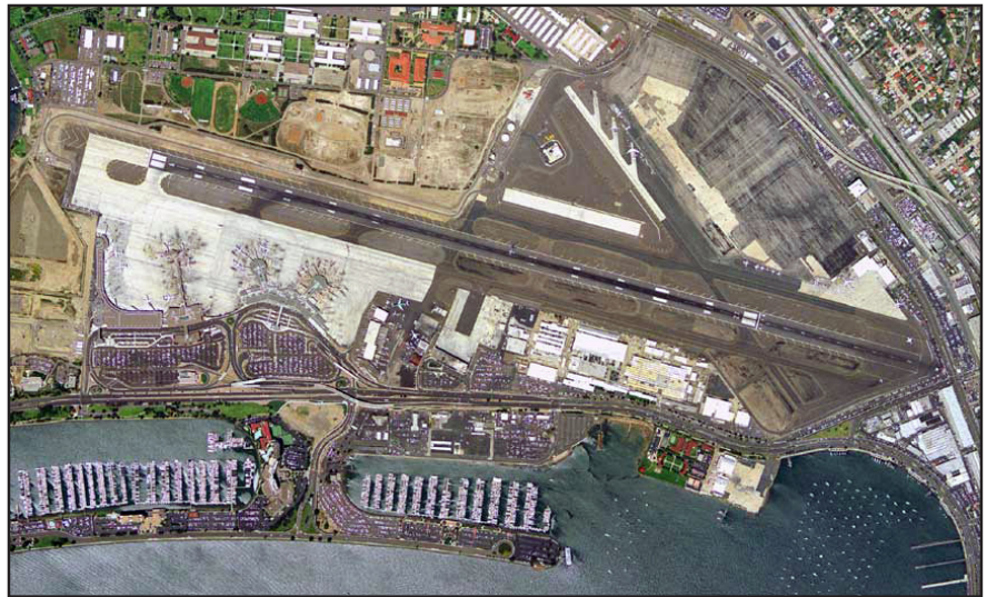
Figure 1: Aerial Photograph of San Diego International Airport
