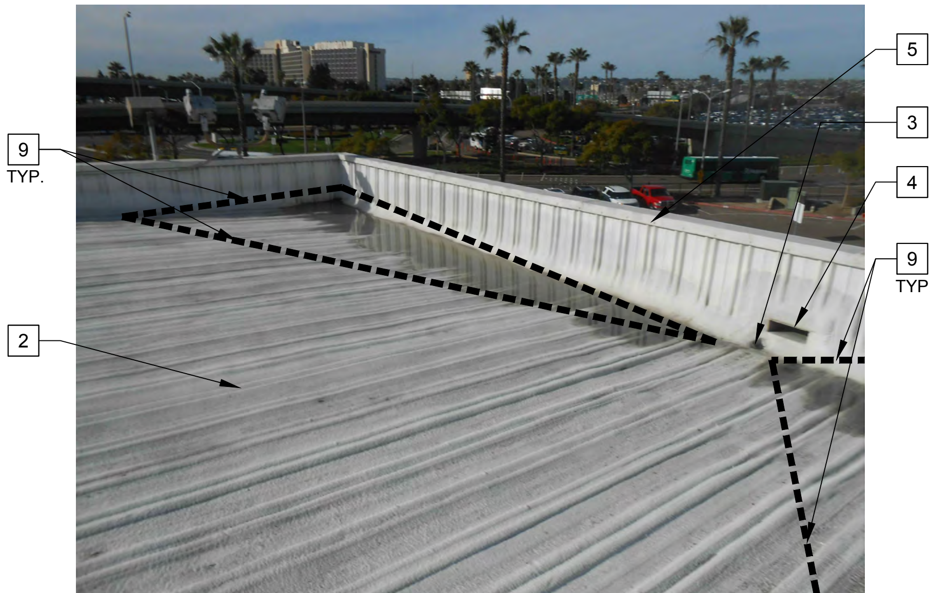
ROOF REFERENCE PHOTO
