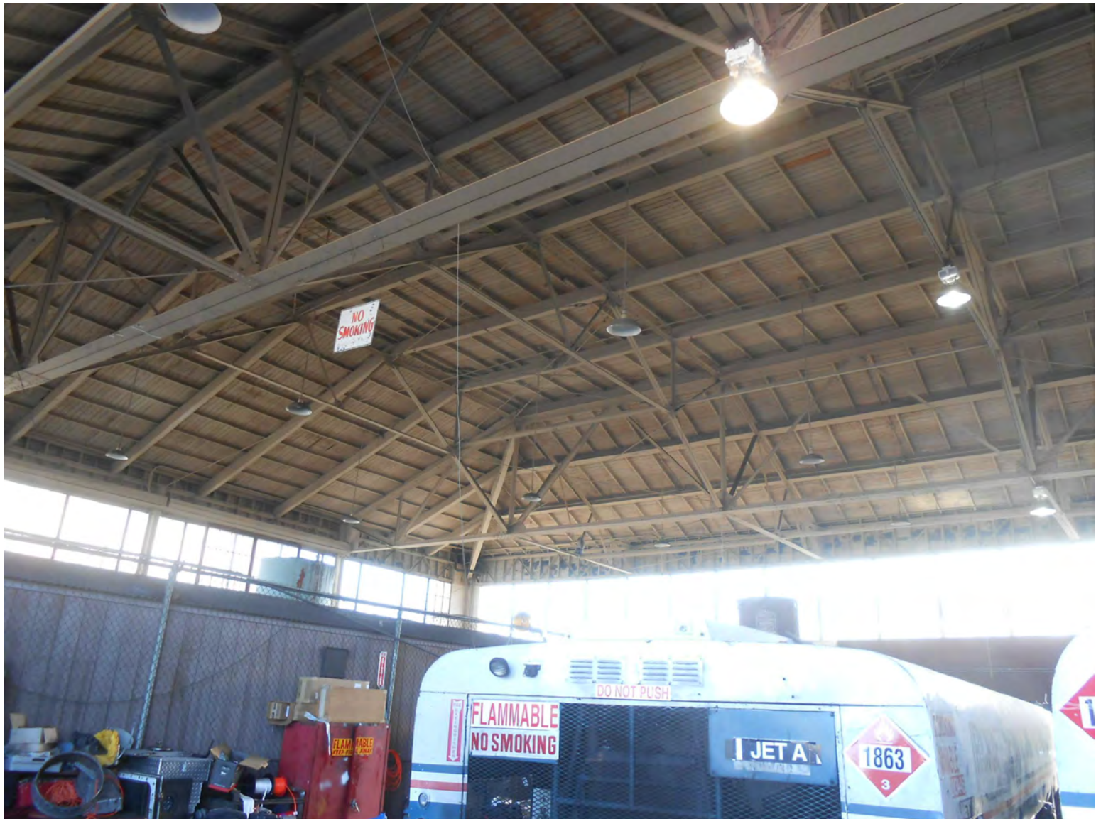
ROOF (INTERIOR) REFERENCE PHOTO
