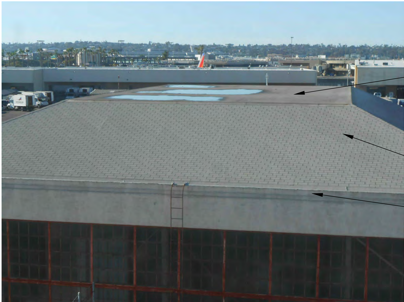
ROOF REFERENCE PHOTO
