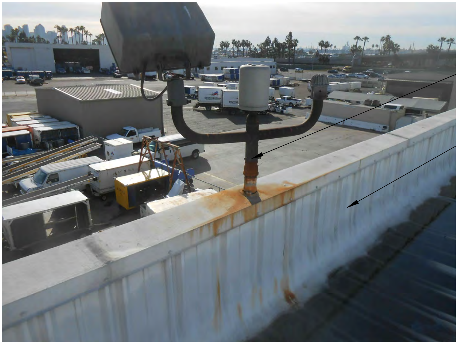
ROOF REFERENCE PHOTO
