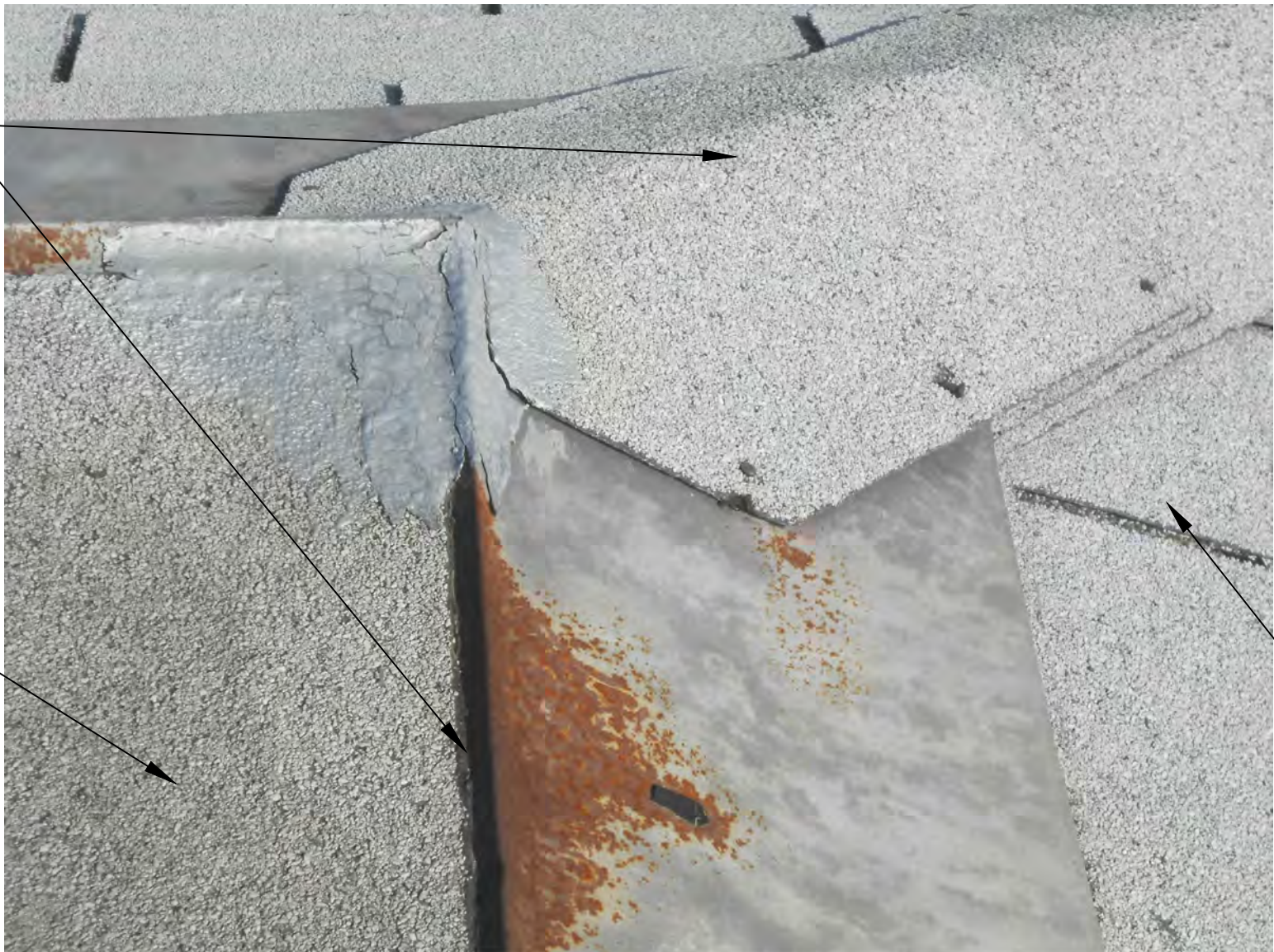
ROOF REFERENCE PHOTO
