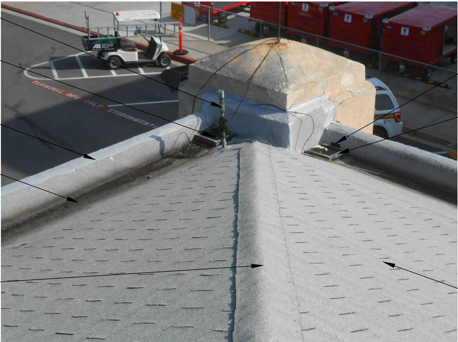
ROOF REFERENCE PHOTO
