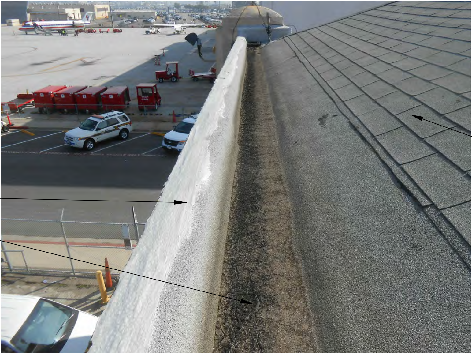
ROOF REFERENCE PHOTO
