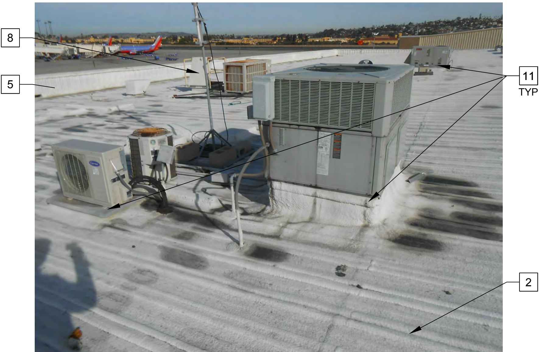
ROOF REFERENCE PHOTO
