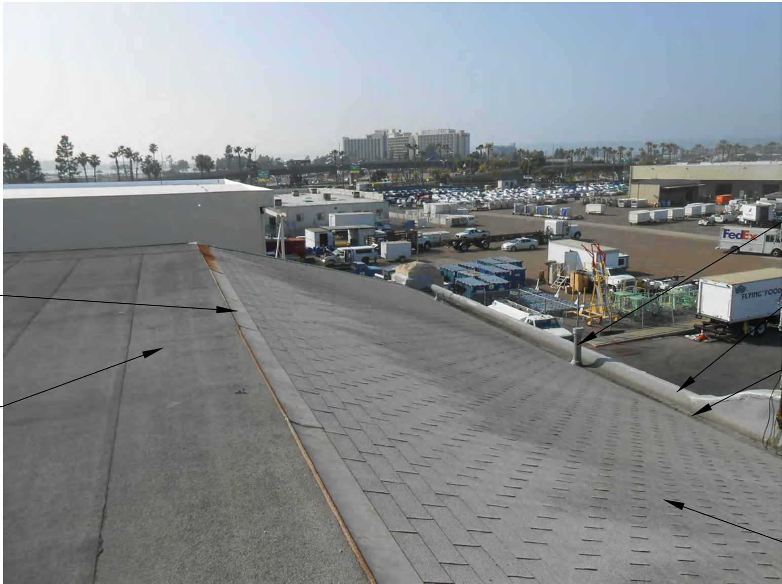
ROOF REFERENCE PHOTO
