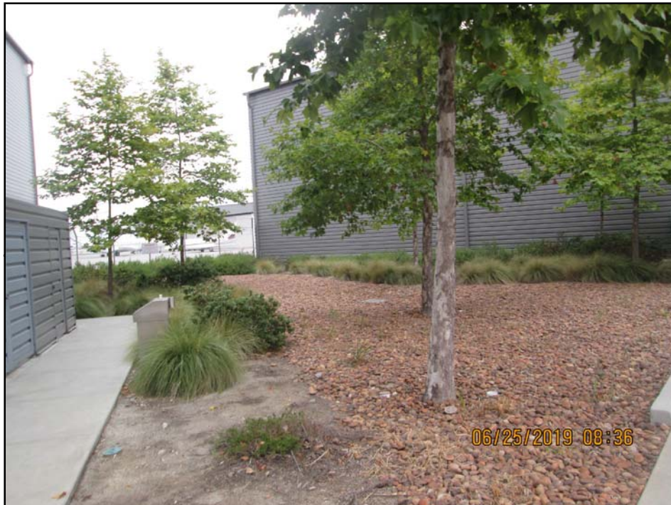
Photo 6. Another example of a maintained stormwater bioswale at SDIA.
