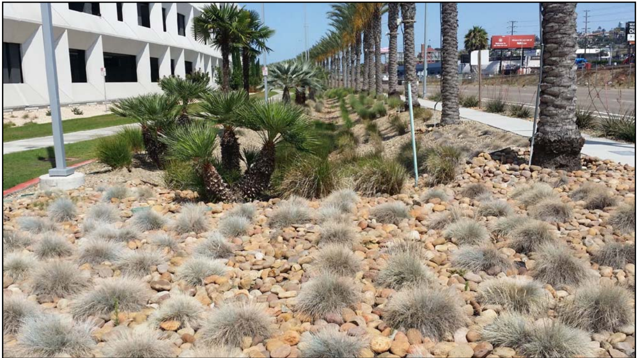
Photo 3. Example of a maintained stormwater bioretention basin at SDIA.
