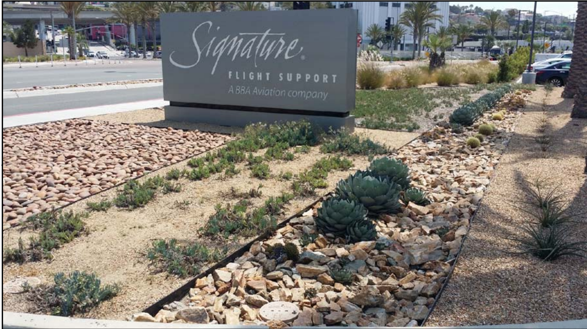
Photo 5. Example of a maintained stormwater bioswale at SDIA.
