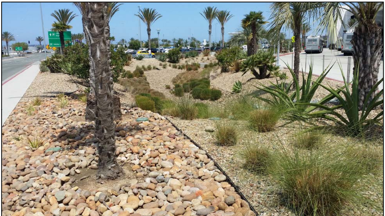
Photo 4. Another example of a maintained stormwater bioretention basin at SDIA.
