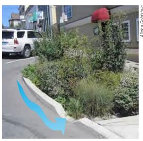
**Figure 4-6.** A curb cut with 45-degree chamfered edges conveys stormwater into a roadside rain garden in Friday Harbor, San Juan Island, WA.
