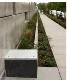
Roof downspout is directed into a stormwater planter in Emeryville, CA.
