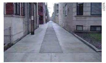
Pervious concrete trench in the center of an alley, Chicago, IL.
