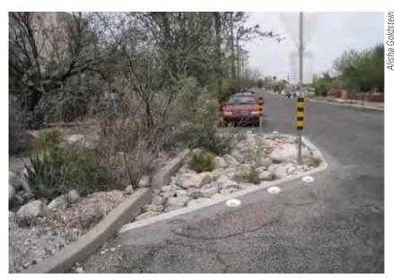
Black and yellow-striped bollards placed around a stormwater curb extension ensures safety for motorists in Tucson, AZ.
