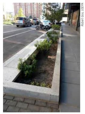
Stormwater planters in Washington, DC, are designed in a series to collect and treat road runoff while allowing adequate pedestrian access to the street and sidewalk.
