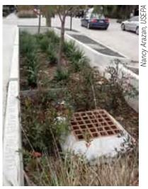
**Figure 4-19.** Raised overflow structure in a bioretention feature in Houston, TX.
