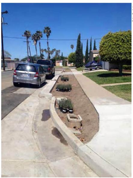
In preparation for planting local native vegetation, a soil media mix was chosen and backfilled into this roadside bioretention area in San Diego, CA.
