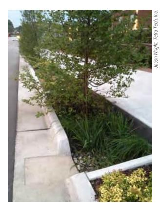
Roadside bioswale with curb-cut inlet in Greensboro, NC.
