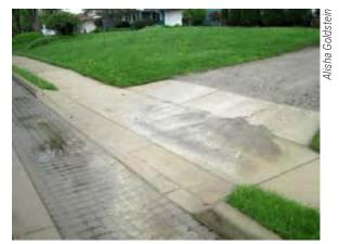
These permeable pavers received runoff from a gravel driveway and became clogged with sediment.
