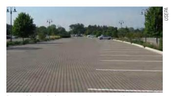
Permeable interlocking concrete pavement, Chicago, IL.
