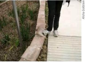
These unsecured blocks installed next to a bioretention area pose a safety risk.
