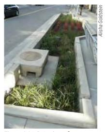
**Figure 4-21.** Raised overflow drain allows a design volume of stormwater to collect in a bioretention area in Portland, OR.
