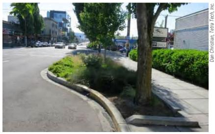
Stormwater curb extensions, such as this one in Portland, OR, capture pollutants such as total suspended solids, total phosphorus, zinc and lead.
