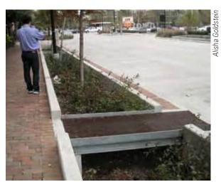
**Figure 4-31.** A grated walkway bridge allows pedestrians to access parked cars on Bagby Street in Houston, TX.
