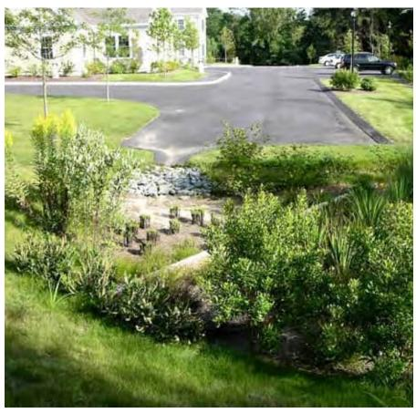
A sediment forebay provides pretreatment for a bioretention cell in Barnstable, MA.
