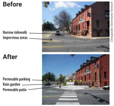
**Figure 2-16.** A roadway was reconfigured to replace a turn lane with green infrastructure practices in Lancaster, PA.
