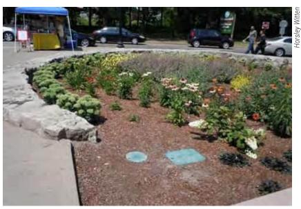
Bioretention in sidewalk with protective stone wall that doubles as a bench in Washington, DC.
