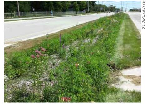
A bioretention area located in the median of an arterial road captures runoff in the Great Lakes region.
