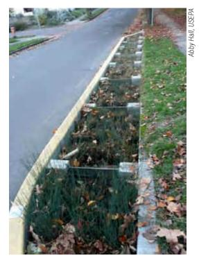
**Figure 4-17.** Concrete check dams slow flow in a stormwater curb extension with a 4.2% slope in Portland, OR.
