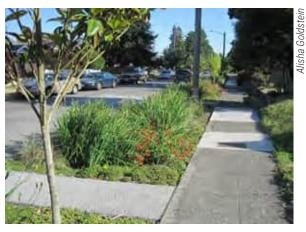
**Figure 4-29.** Permeable pavement walkways provide access to on-street parking in Seattle, WA.
