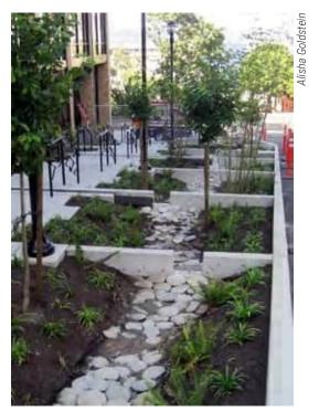
**Figure 4-18.** Concrete check dams with splashpads slow flow velocities along a steep slope in Seattle, WA.
