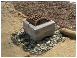
The large-spaced grate on this overflow drain will not prevent floatables and debris from entering.
