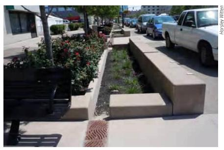
Interconnected stormwater planters include protective walls alongside the parking lane in Niagara Falls, NY.
