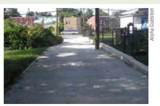
Permeable concrete installed in a Washington, DC, alley.
