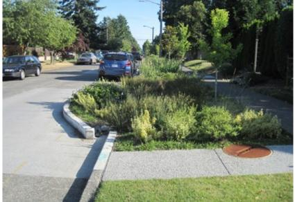
Parking impacts minimized by using a mid-street stormwater curb extension in
