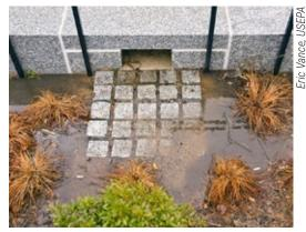
**Figure 4-15.** Concrete paver splashpad dissipates energy from stormwater entering from a trench in Washington, DC.
