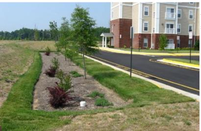
Vegetated filter strip at the edge of a parking lot intercepts and filters stormwater runoff before the water reaches the infiltration bed at the center of the practice.
