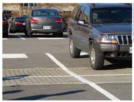
Permeable pavers installed at the downgradient end of parking bays collect surface runoff and allow it to infiltrate.
