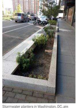
Stormwater planters in Washington, DC, are designed in a series to collect and treat road runoff while allowing adequate pedestrian access to the street and sidewalk.
