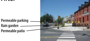
Figure 2-16. A roadway was reconfigured to replace a turn lane with green infrastructure practices in Lancaster, PA.
