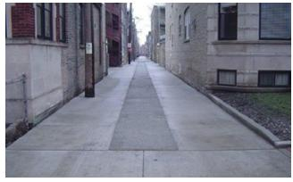
Pervious concrete trench in the center of an alley, Chicago, IL.
