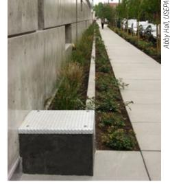
A stormwater planter can be designed to capture and treat roof runoff.
