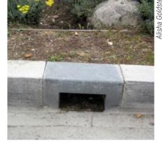
This undersized curb cut is easily clogged by mulch and other debris.
