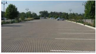
Permeable interlocking concrete pavement, Chicago, IL.
