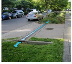
**Figure 4-9.** Trench-grated drain conveys stormwater between swales while also capturing runoff in Seattle, WA.
