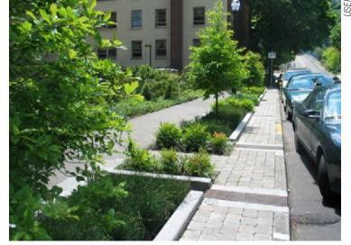
Sidewalk planters are equipped with bridges to provides access to parking areas in Seattle, WA.
