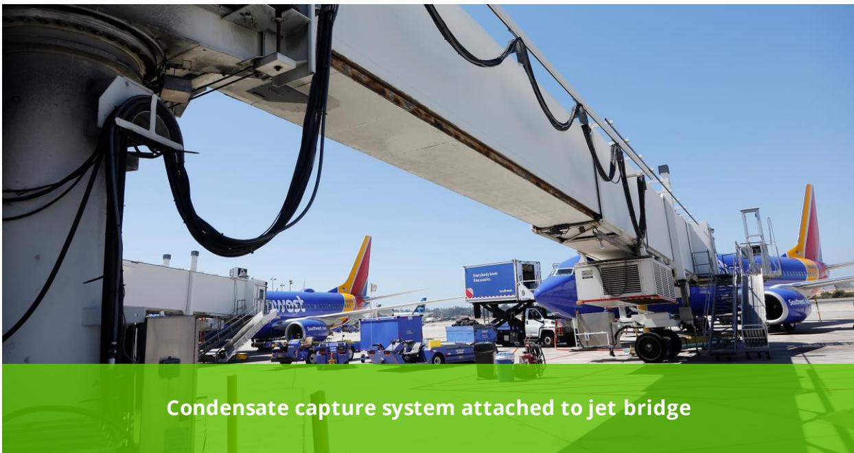
Condensate capture system attached to jet bridge
