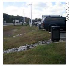
These trash cans, installed in front of stormwater inlets, block flow.
