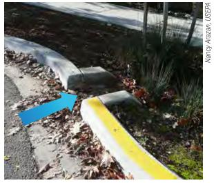
**Figure 4-7.** A curb cut with wings retains the side slope grade and directs street runoff into a bioretention feature in Portland, OR.
