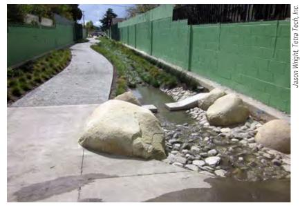
**Figure 4-14.** A sediment forebay with weir helps trap sediment and control flow volume in an alleyway bioswale in Los Angeles, CA.
