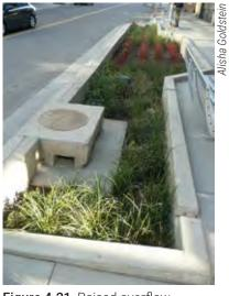
**Figure 4-21.** Raised overflow drain allows a design volume of stormwater to collect in a bioretention area in Portland, OR.
