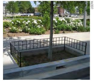
**Figure 4-35.** Short fencing protects pedestrians from stepping into this stormwater tree box in Washington, DC.
