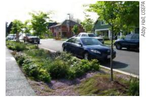
Bioswale next to a permeable pavement sidewalk in Seattle, WA.
