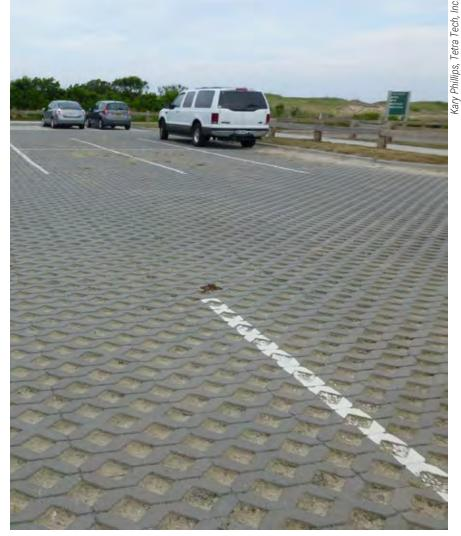
Sand-filled permeable pavers allow rainfall to infiltrate instead of generating erosive runoff in a sensitive coastal area in Virginia Beach, VA.
