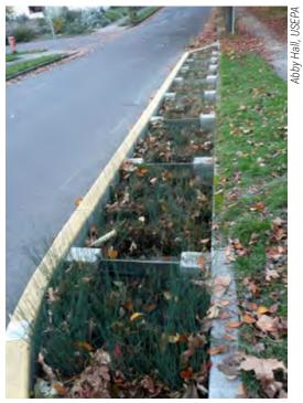
**Figure 4-17.** Concrete check dams slow flow in a stormwater curb extension with a 4.2% slope in Portland, OR.
