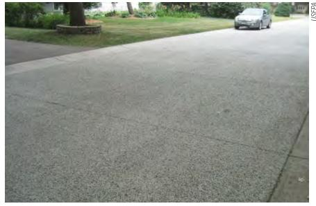
Pervious concrete pavement on a low-speed residential roadway in Shoreview, MN.
