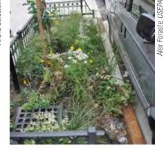
This stormwater planter does not provide space for passenger exit.
