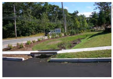
Roadside bioretention area includes a sidewalk bridge over the inlet to avoid obstructing pedestrian flow.
