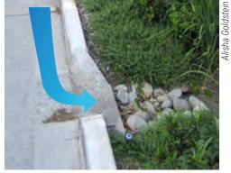
**Figure 4-2.** An angled curb cut with a graded gutter, Seattle, WA.
