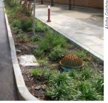
The overflow drain is placed in the flow path of water entering the practice.
