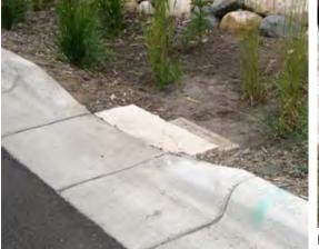
**Figure 4-26.** A wide-angled curb cut with an energydissipating splashpad also serves as access steps for maintenance in Maplewood, MN.
