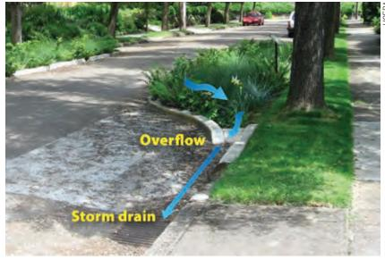
Runoff enters the upper end of this curb extension, and the overflow volume exits through an opening on the lower end and drops into a storm drain.
