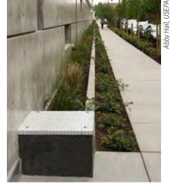
A stormwater planter can be designed to capture and treat roof runoff.
