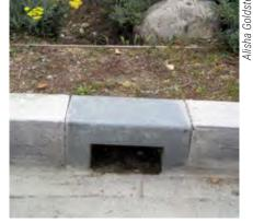
This undersized curb cut is easily clogged by mulch and other debris.
