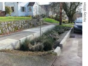
Curb cuts in the sidewalk and street allow for runoff to flow into this stormwater planter in Portland, OR.
