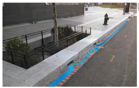
**Figure 4-23.** In this tree pit bypass system in Washington, DC, curb cuts allow stormwater to enter until the practice is filled, at which point additional flow bypasses the system and continues down the street to the storm drain.
