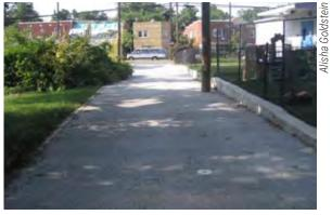
Permeable concrete installed in a Washington, DC, alley.
