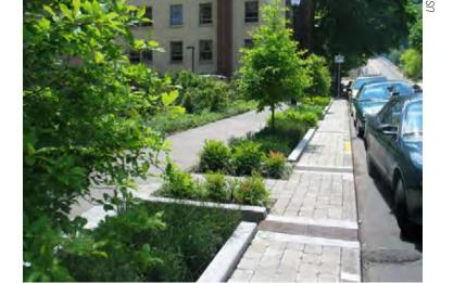
Sidewalk planters are equipped with bridges to provides access to parking areas in Seattle, WA.
