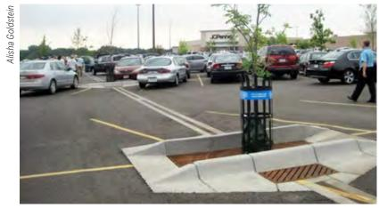
Trees are planted in groves connected by trenches in this parking lot at the Maplewood Mall, MN. Tree trenches extend 8 to 12 feet wide and 4 feet deep for a total of 1 mile in length. Angled curbs were designed to allow snow plows to roll smoothly over them.
