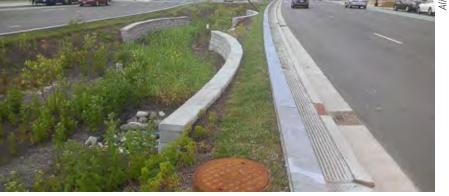
Medians with rain gardens manage stormwater runoff from the street collected via stormwater inlets connected to subsurface pipes in Arlington, VA.
