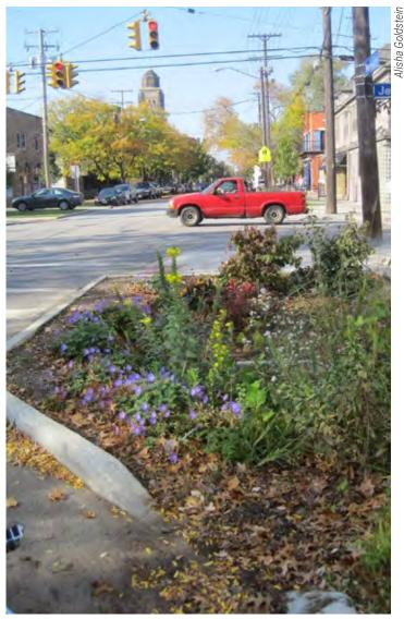
Traffic calming and stormwater bioretention curb bump-out project, Cleveland, OH.
