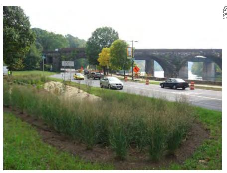
A bioretention area is located adjacent to an arterial road along the Schuylkill River in Philadelphia, PA.
