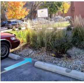
**Figure 4-5.** The space between adjacent wheel stops allows stormwater runoff to enter a vegetated swale in a parking lot in Cleveland, OH.
