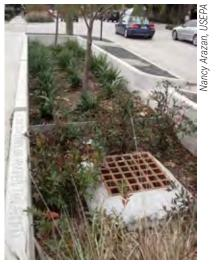
**Figure 4-19.** Raised overflow structure in a bioretention feature in Houston, TX.
