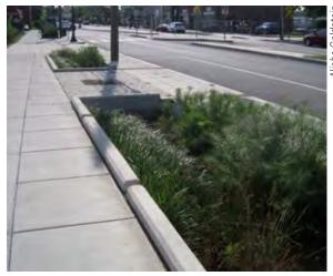
**Figure 4-33.** A raised curb with inlets defines the edges of a sidewalk stormwater planter in Washington, DC.
