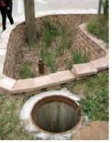
**Figure 4-27.** To facilitate maintenance, an observation well is installed next to a bioretention area in Houston, TX.
