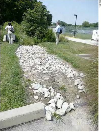
A sediment forebay provides pretreatment for parking lot runoff entering a bioretention cell at Villanova University, PA.
