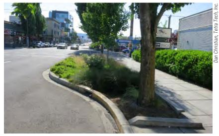
Stormwater curb extensions, such as this one in Portland, OR, capture pollutants such as total suspended solids, total phosphorus, zinc and lead.
