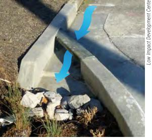
**Figure 4-4.** Metal extension inlet structure provides a wide opening for stormwater flow to enter the stormwater feature.
