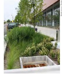
**Figure 4-20.** Concrete band constructed around the outflow allows ponding in Nashville, TN.
