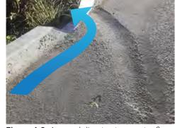
Figure 4-3. A runnel directs stormwater flow, San Juan Island, WA.
