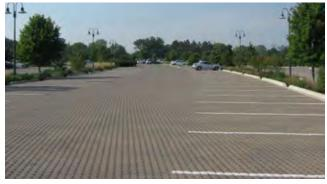
Permeable interlocking concrete pavement, Chicago, IL.
