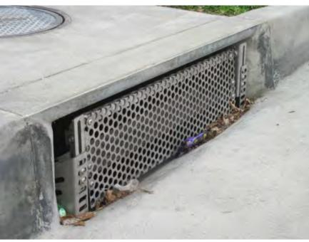
A curb inlet cover allow runoff to enter a catch basin but prevents inflow of trash.
