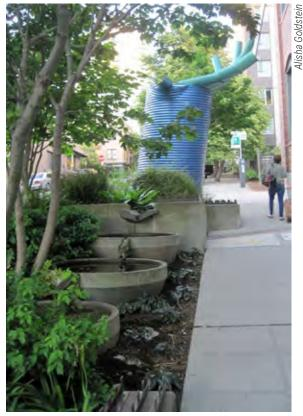
The Beckoning Cistern serves as an artistic feature and a stormwater management practice. Designed to resemble a large upturned hand, the 15-foot-tall structure adds visual interest while collecting roof runoff, some of which is directed into a series of cascading stormwater planters along Vine Street in Seattle, WA.
