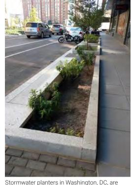
designed in a series to collect and treat road runoff while allowing adequate pedestrian access to the street and sidewalk.
