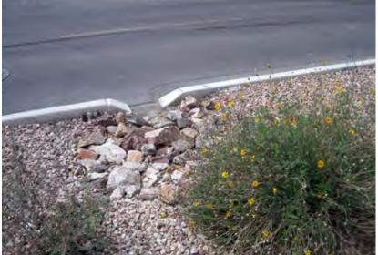
**Figure 4-13.** A sediment forebay slows the concentrated flow to allow sediment to drop out of suspension in Tucson, AZ.
