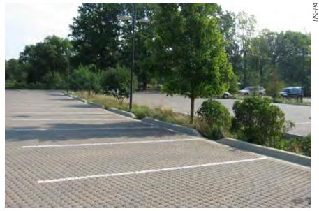
**Figure 4-24.** Vegetated swales were installed adjacent to a permeable parking lot in Chicago, IL, to provide overflow control and back-up infiltration as needed.
