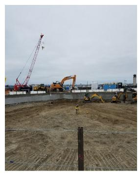
Start of second level of excavation – before reaching groundwater
