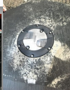
TYPICAL RE-INSTALLED IN-PAVEMENT EDGE LIGHT MATERIALS
