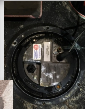
TYPICAL RE-INSTALLED IN-PAVEMENT EDGE LIGHT MATERIALS
