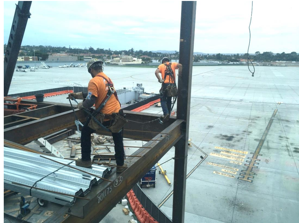
Metal Floor Decking Installation
