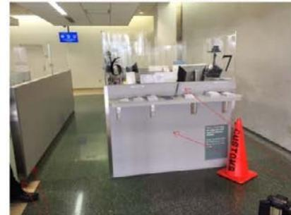
INSTALL FULL HEIGHT STAINLESS STEEL WAINSCOT ON ALL DIVIDING WALLS (TYP. @ 2ND FLOOR BOOTHS)
