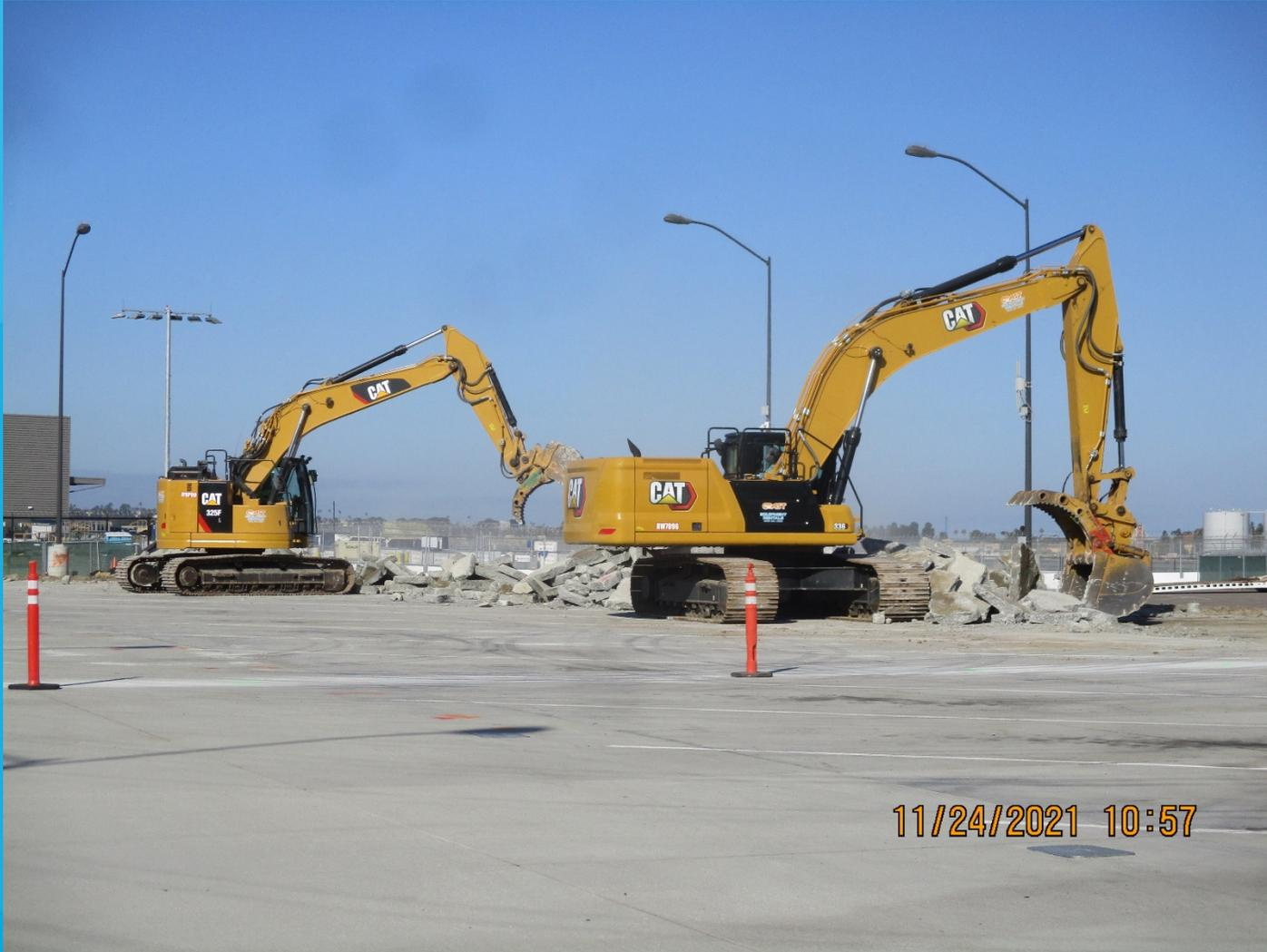
Demolishing RCC Bus Parking Slab
