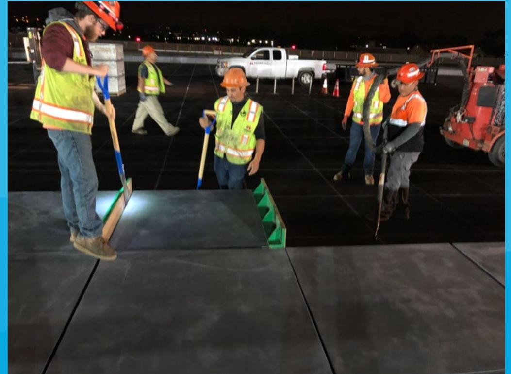
Adjusting New EMAS Block Spacing
