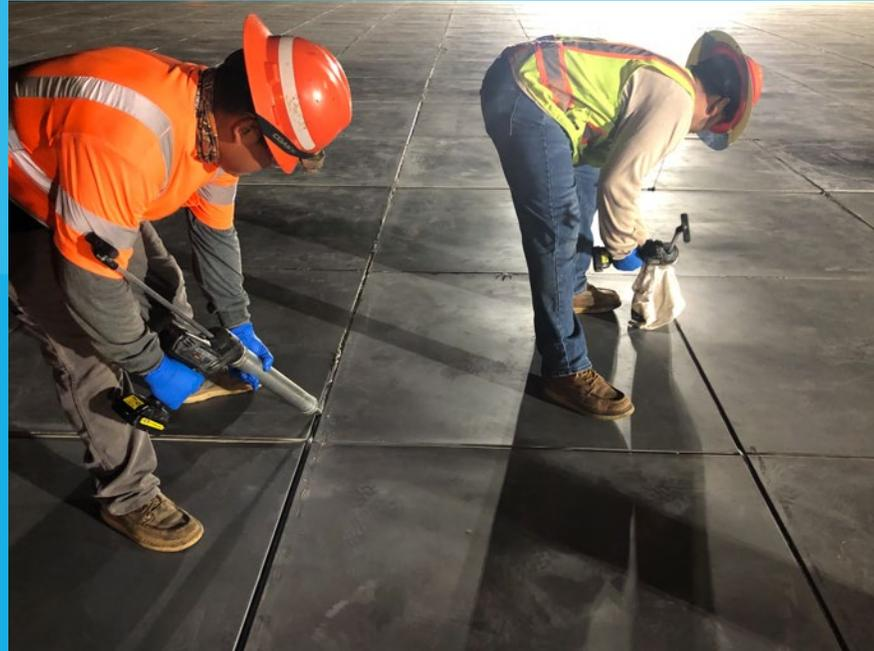
Sealing Joints between EMAS Blocks
