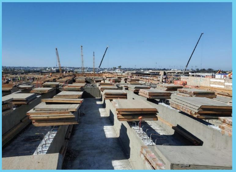
Elevated Roadway after forms are stripped from first concrete placement
