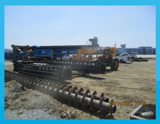
Unloading pile drilling equipment
