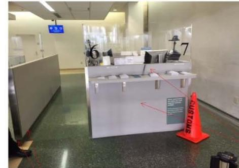
INSTALL FULL HIGHT STAINLESS STEEL WAINSCOT ON ALL DIVIDING WALLS (TYP. @ 2ND FLOOR BOOTHS).
