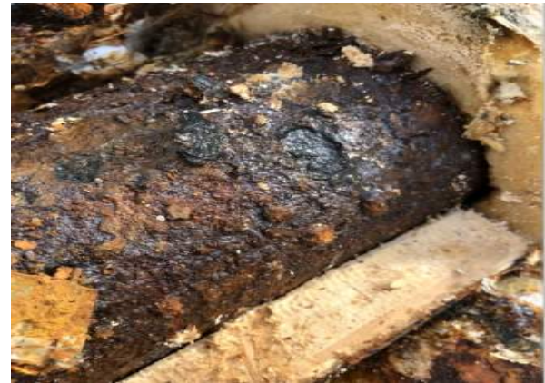
la Metal Jacket Damage & Corrosion
