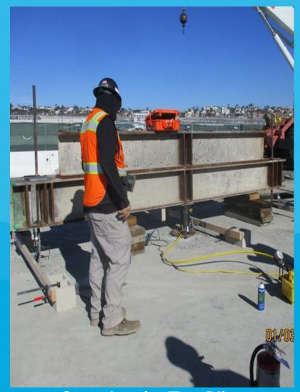
Stressing the Test Pile
