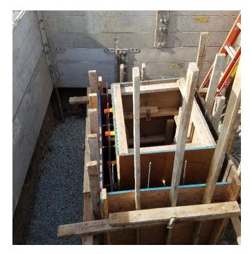
Concrete forms in place for one of many drainage structures to be poured at the ASB site
