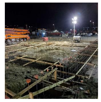
Steel reinforcement being placed before pour of concrete grade beams
