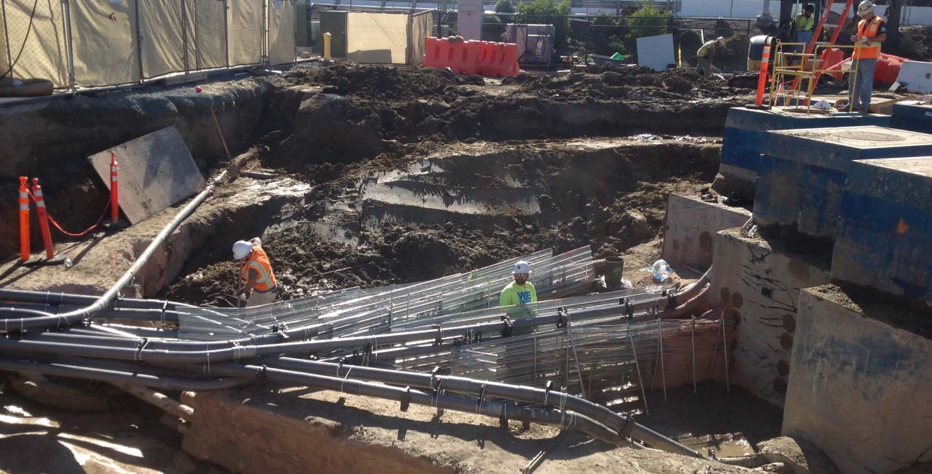
Relocation of Primary 12kv Electrical Ductbanks
