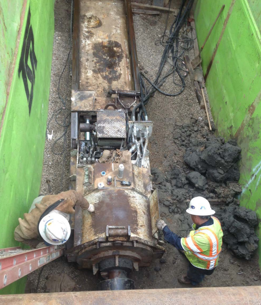
Preparation of Jack & Bore Rig
