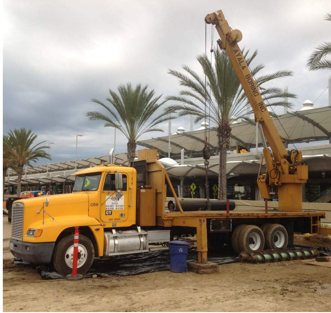
Lowering Pipe Casing into Jack & Bore Pit 7
