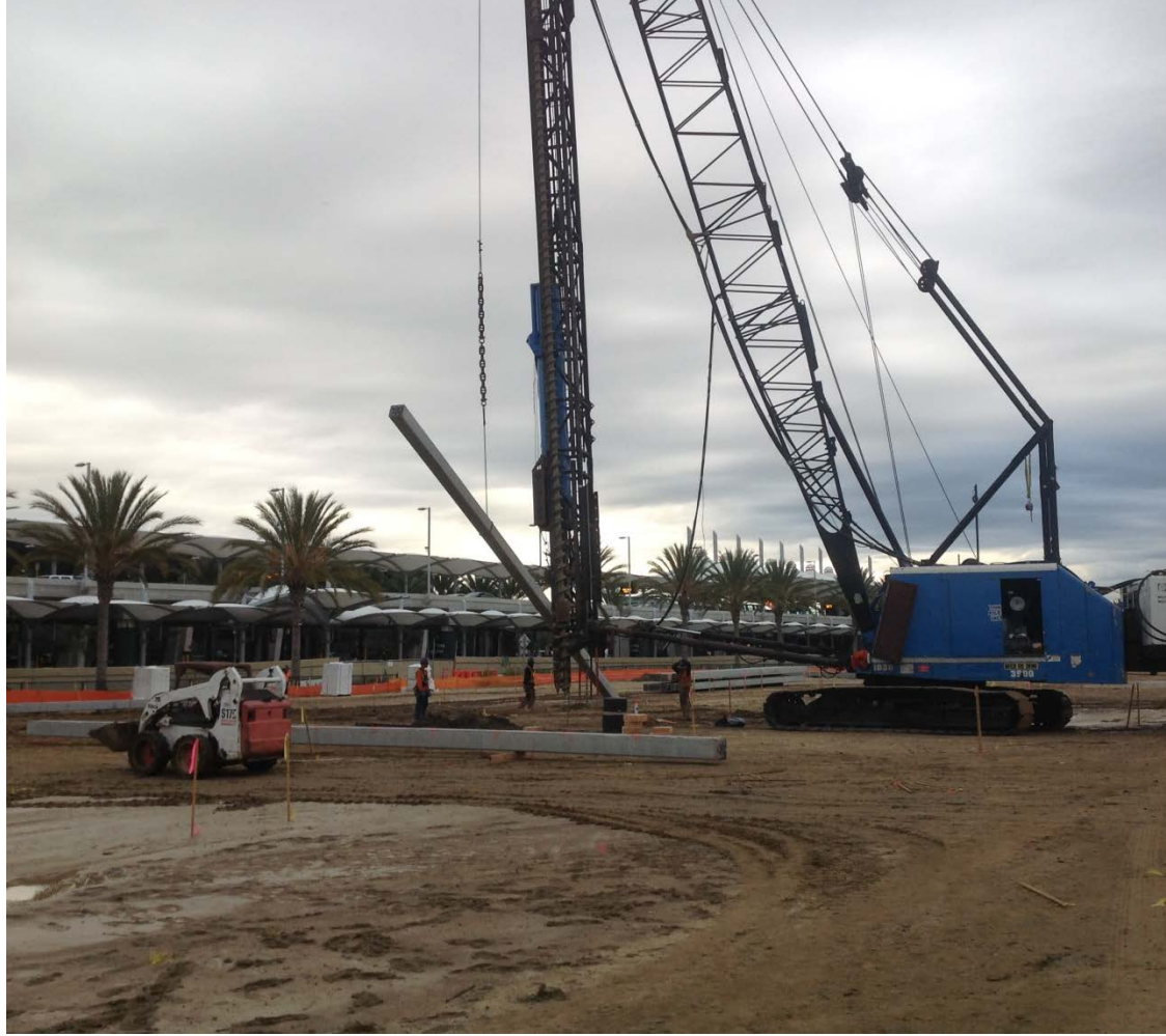
Lifting Pile to Place into Driving Rig
