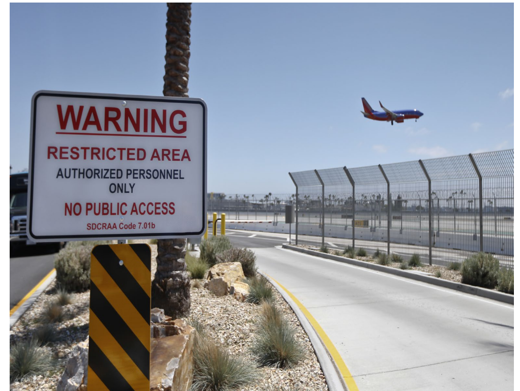
Example of Perimeter Fencing
