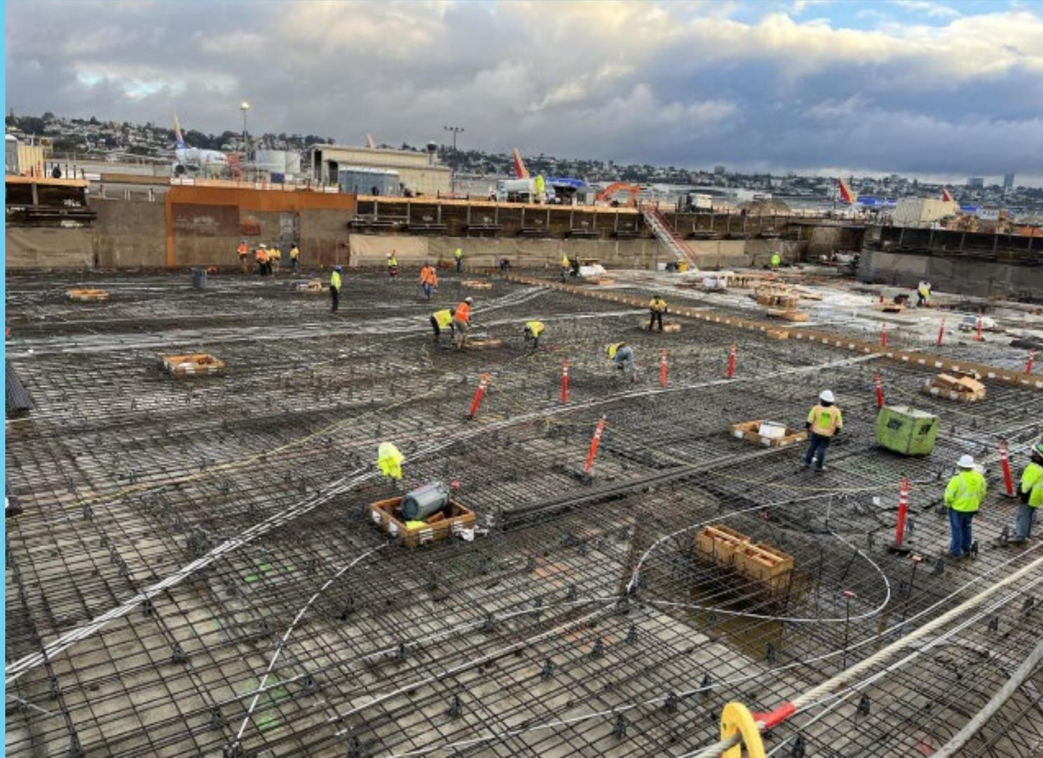
Rebar and conduit before a concrete placement in the CBIS
