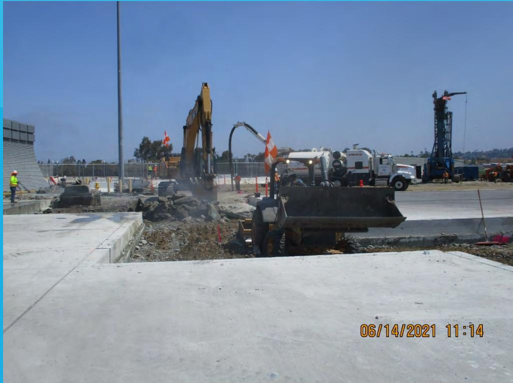
Demolishing concrete apron
