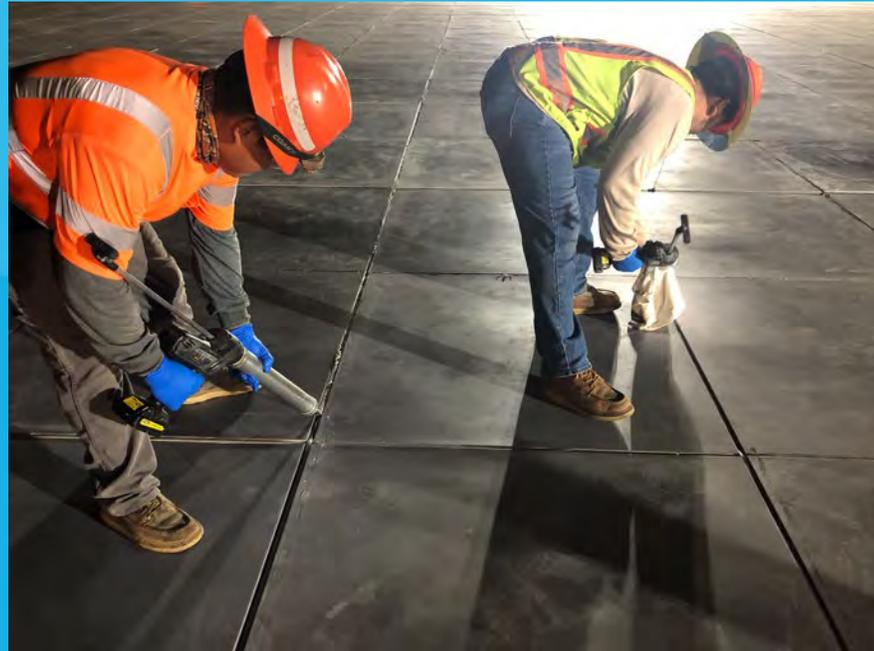
Sealing Joints between EMAS Blocks
