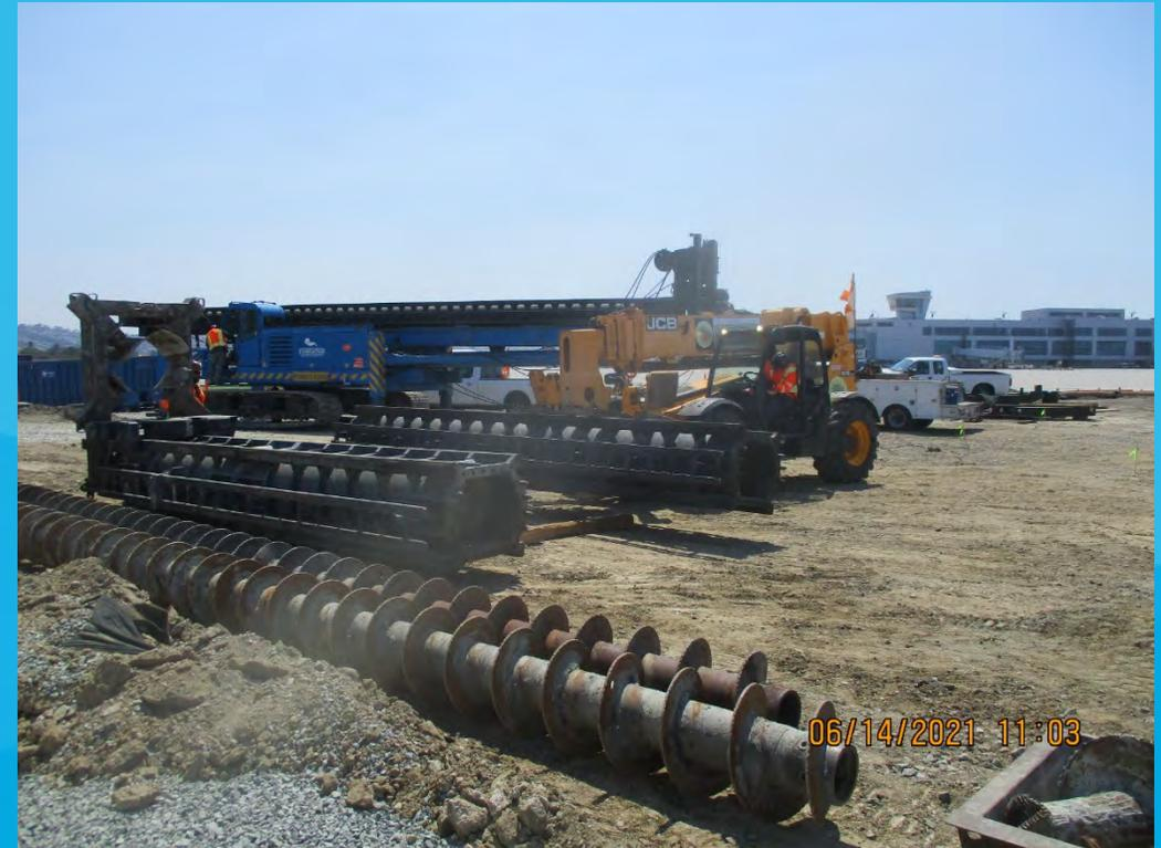
Unloading pile drilling equipment
