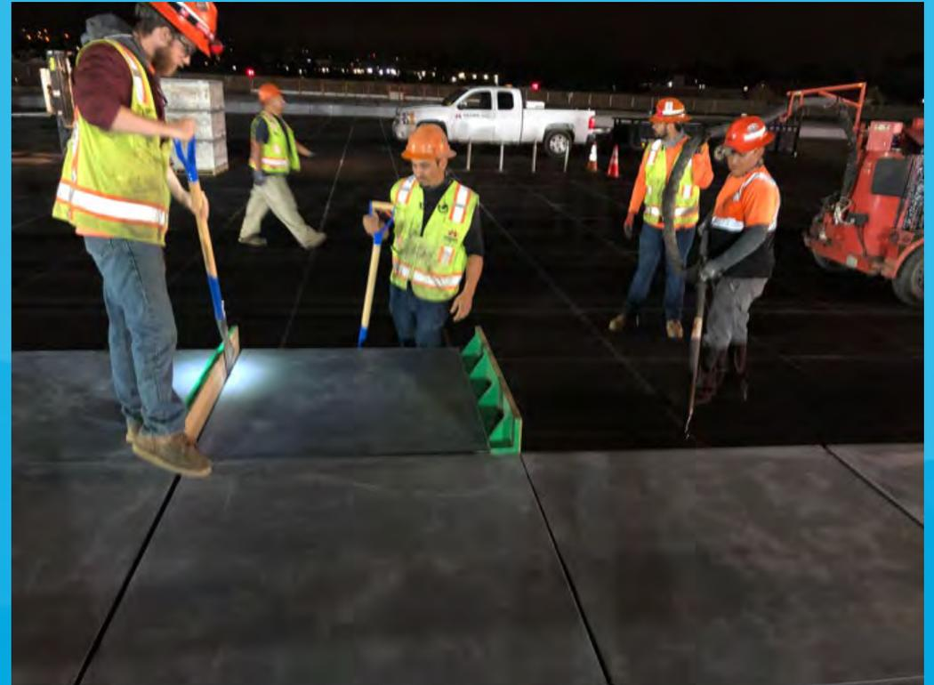
Adjusting New EMAS Block Spacing
