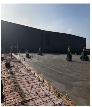
Finishing the floor slab over the vapor containment barrier at the FMD Shops building
