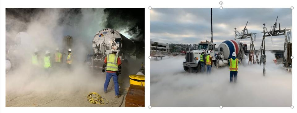
Liquid Nitrogen Being Injected Into Concrete Mixing Trucks on Site
