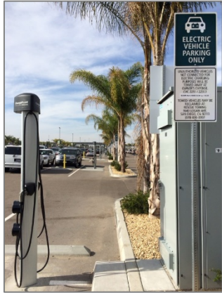
Expand EV Charging & Parking
