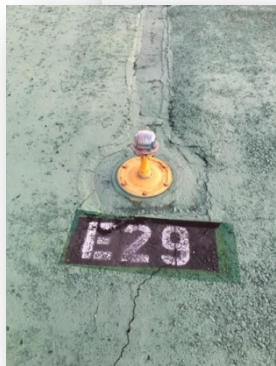
TYPICAL RE-INSTALLED ELEVATED EDGE LIGHT MATERIALS
