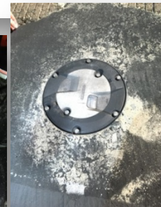
TYPICAL RE-INSTALLED IN-PAVEMENT EDGE LIGHT MATERIALS
