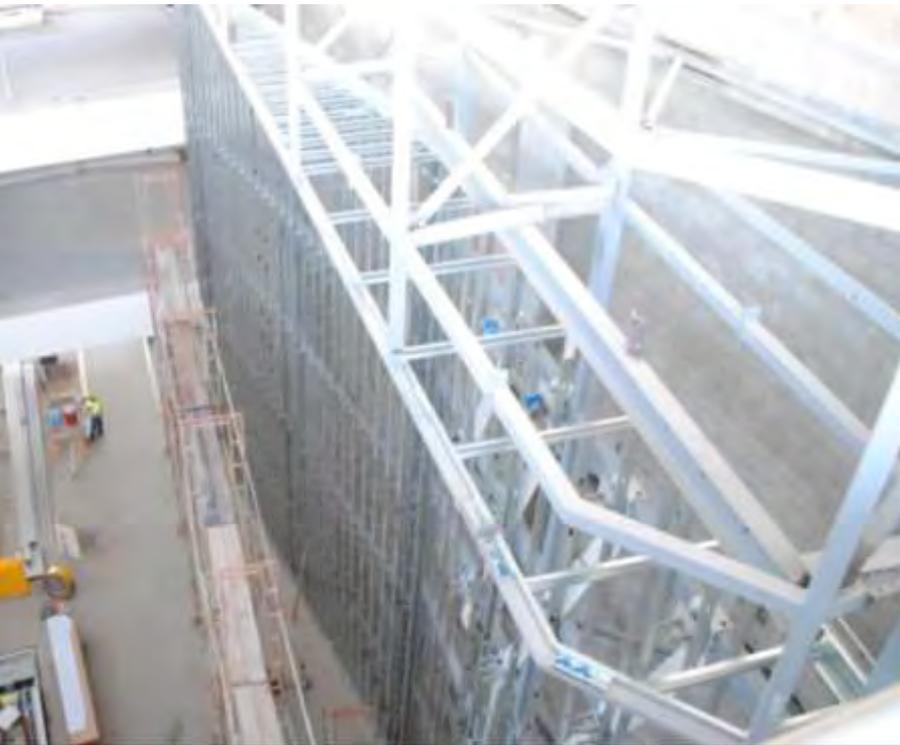
Substructure for Art Wall
