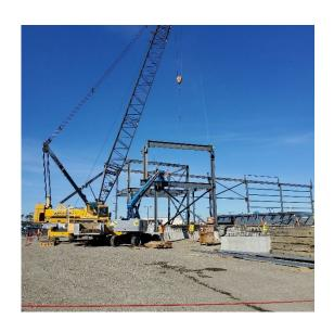
Two 100' high cranes being utilized to erect steel framing as the ASB
