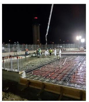
Placing the reinforced concrete floor slab over the vapor containment barrier
