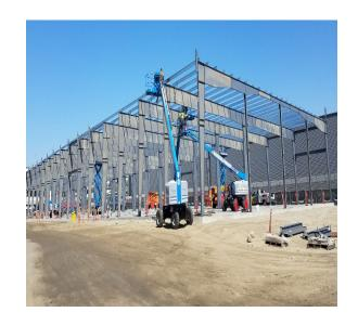
Structural steel erection at FMD Shops building nearly complete
