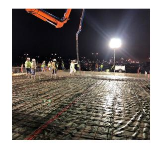
Steel reinforcement in place for the pour of the floor slab
