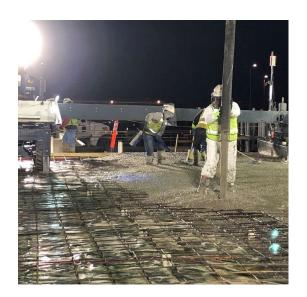
Concrete being pumped and placed for night time pours of the floor slab
