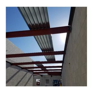
Installation of roof structure utilizing bolting plates
