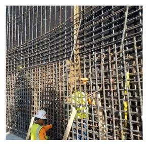
Tons (literally) of steel rebar being placed to allow concrete walls to withstand external pressure without cracking
