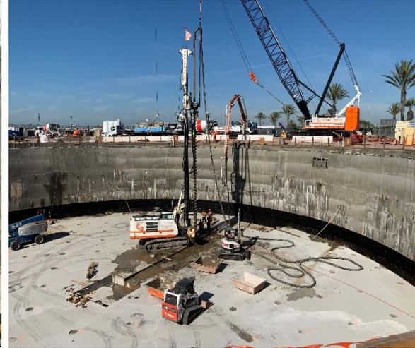
Excavation and Anchor Pile Placement
