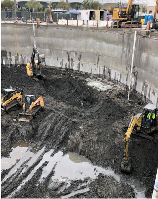
Start of fifth level of excavation – pumps keeping up with groundwater
