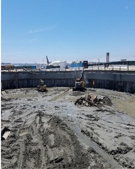
Second level of excavation complete – groundwater encountered at site
