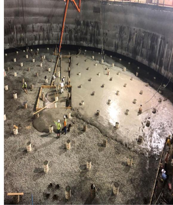
Pouring mud slab after reaching final grade at cistern
