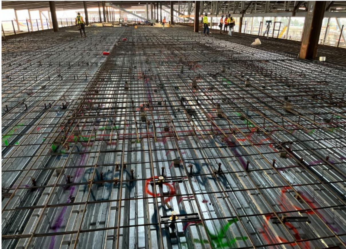
View of Metal Deck & Reinforcing Bars
