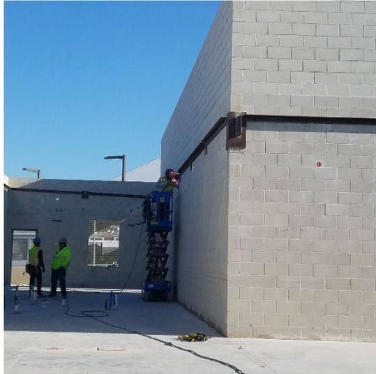
Welding bolting plates for roof
