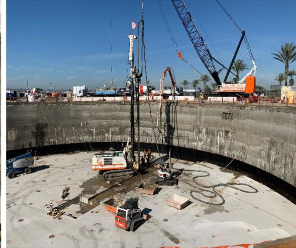
Excavation and Anchor Pile Placement
