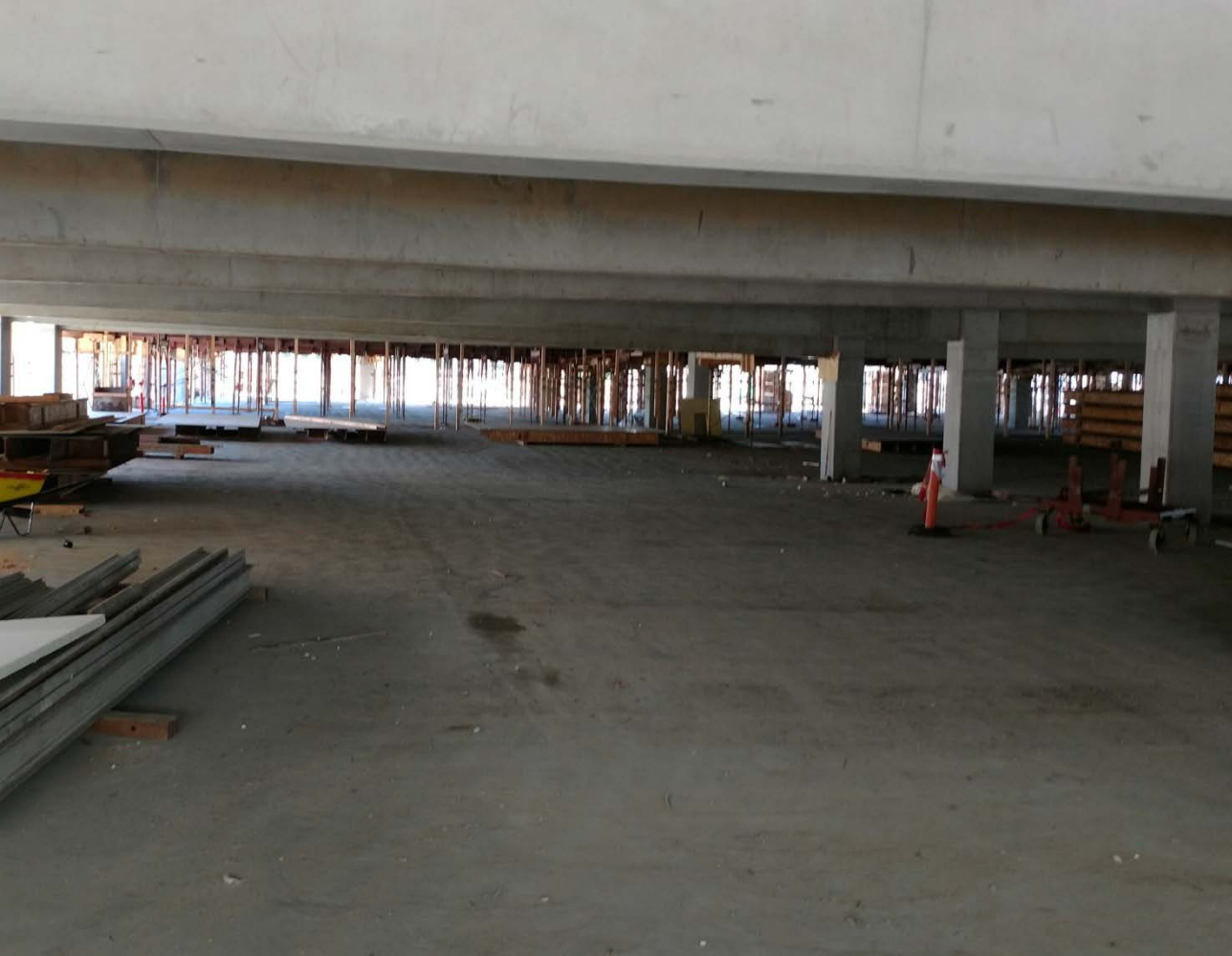
Slab on Grade with 2 nd Floor Elevated Deck Above
