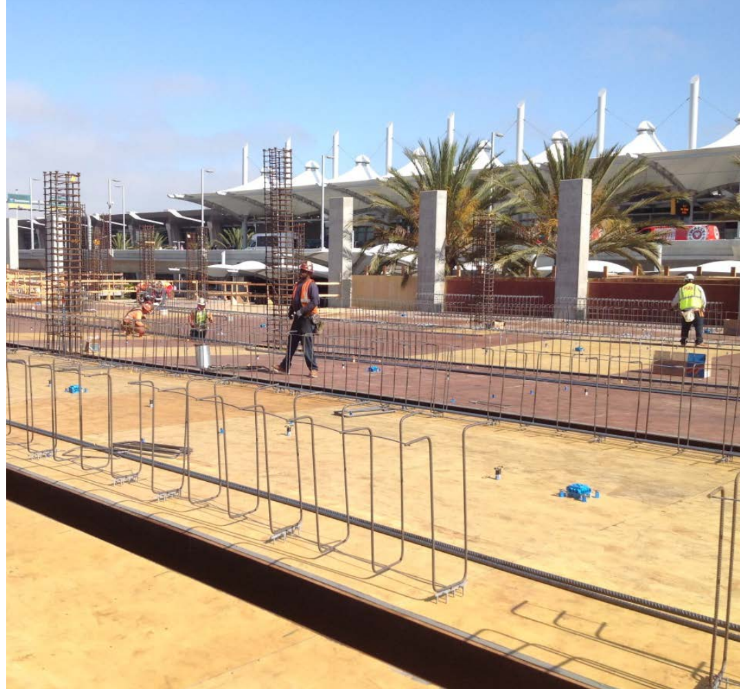
Preparation of 2 nd Level Deck
