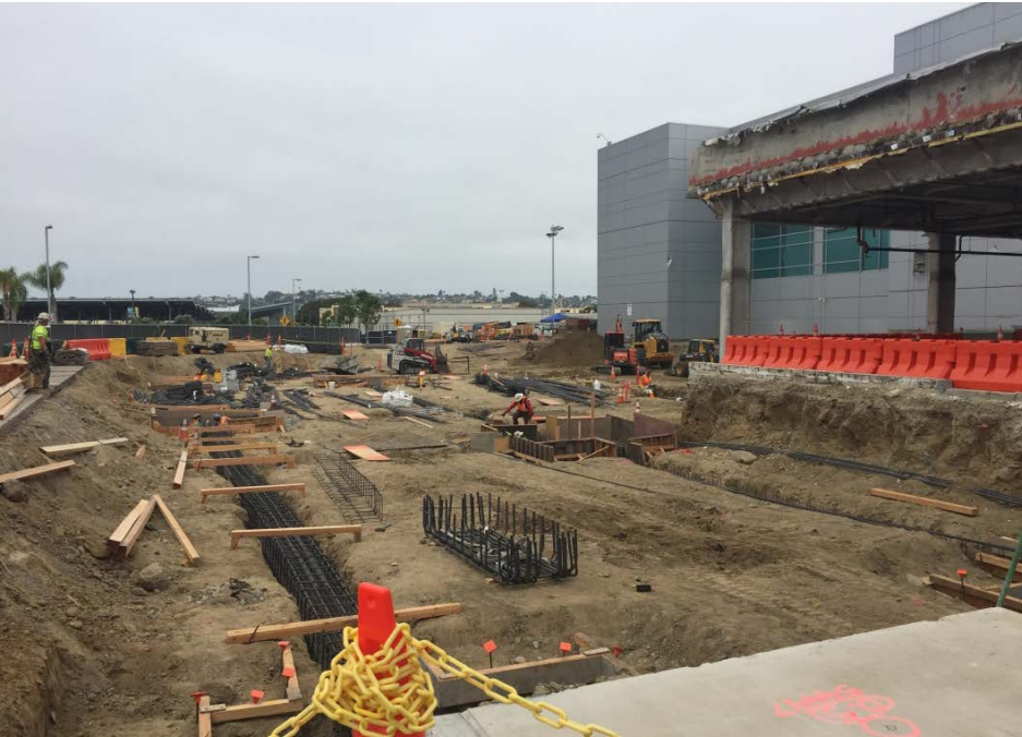
West View: Steel Reinforcement installation for Grade Beams
