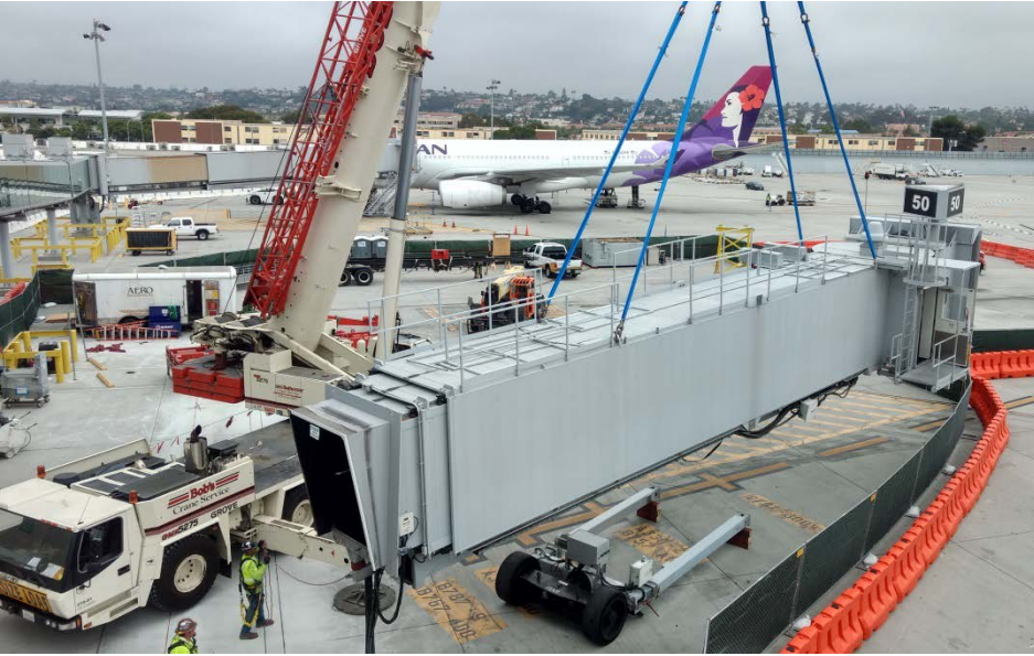
Gate 50 Passenger Boarding Bridge Removal
