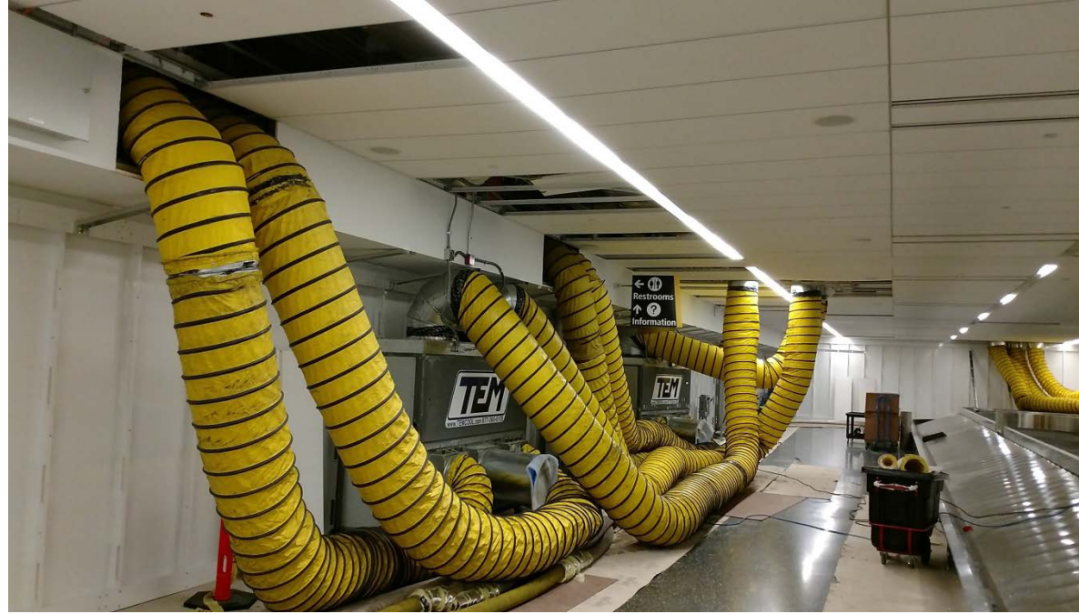
Temporary Cooling System for 1 st Floor T2W During Demolition
