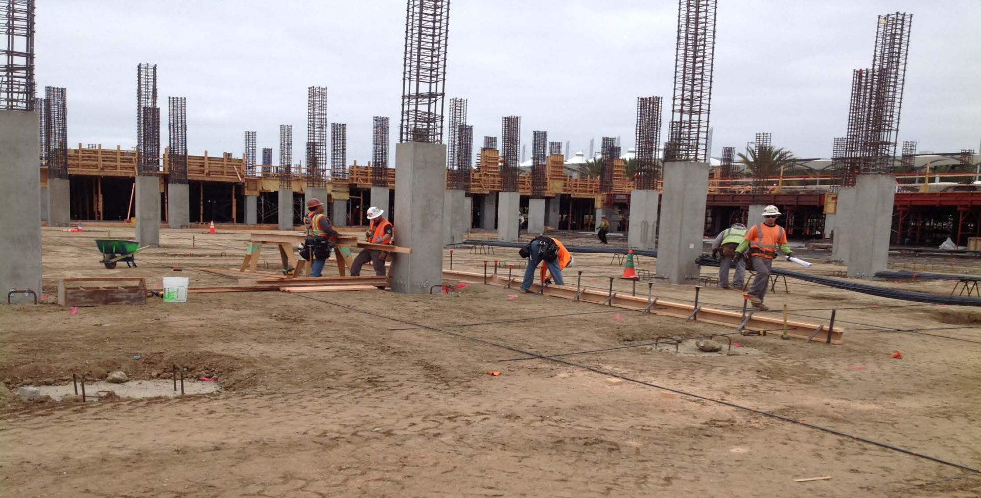
Construction Progress: Preparation of Slab on Grade
