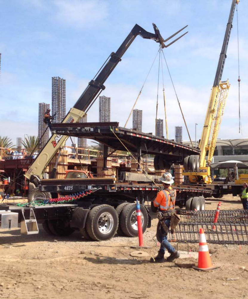
Falsework for 2 nd Level Deck
