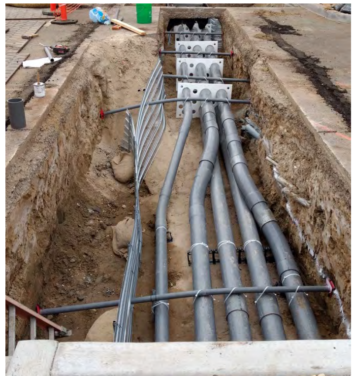
12 KV Relocation—New Ductbanks
